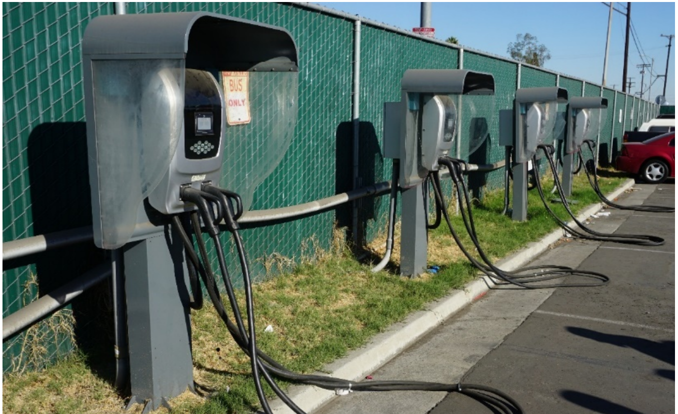
Figure 8: LADOT Depot Chargers
